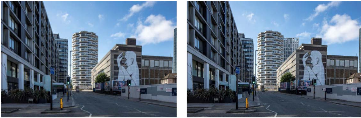
Images 23 and 24: Existing and proposed view from the north of the site along Cherry Orchard Road
